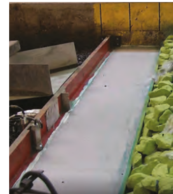
Rock revetment testing, Dungeness
