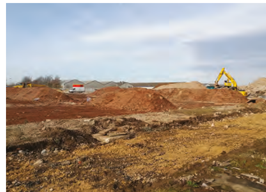
Early earthworks optimisation saves costly movement/disposal
