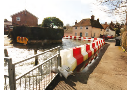
Localised temporary flood defences
